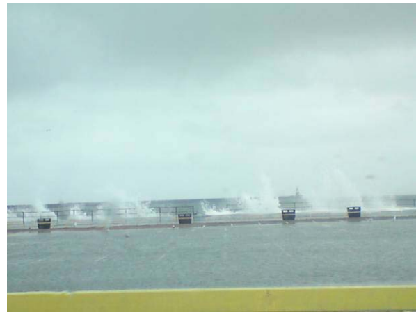
Littlehaven – Sea flooding of hinterland
