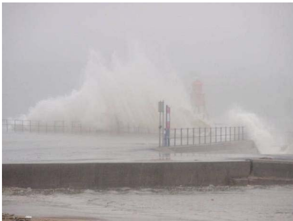
Littlehaven – Violent wave overtopping
